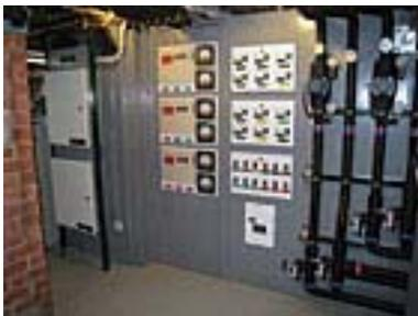
The residence of Brian K. Nelson and family, and the office of NMD Inc., house a unique mechanical room. This view shows DDC panels 1 and 2 on the left, air zone controls in the middle, and variable-speed circulator controls on the right.
