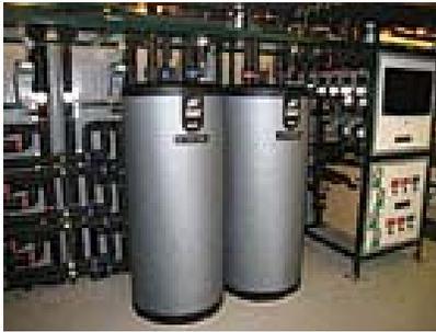
The basement of the Nelson residence is used as the testing grounds for new heating and cooling technologies and control systems. Here, chilled and hot water buffer tanks are on the left, circulators for
