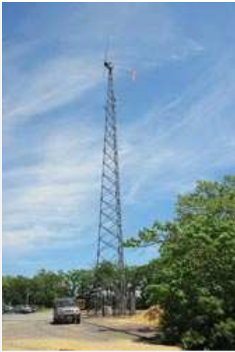
As a reference for gauging the height of wind turbines, the regional high school's tower is 100 ft. tall and the top of the blade tips 112 ft. Photo by Ralph Stewart
