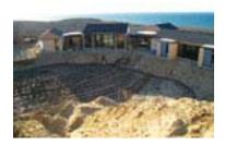
A 10-ton, closed-loop, horizontal geothermal field serves five water-to-air heat pumps (five forced-air zones); one water-to-water heat pump (three radiant floor-warming zones and domestic hot water preheat) in this Martha's Vineyard LEED for Homes residence. (Photo courtesy of NMD.)
