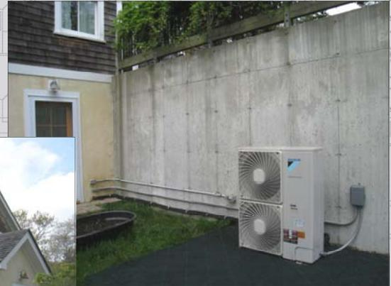
*A 3,000 square foot home with Daikin Altherma as the solution that uses electricity, operates at geothermal efficiency levels of 200 to 400%, has a tiny outside footprint, and heats water for the home's radiant floors and domestic hot water system.*
