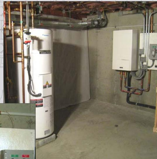
*A Daikin Altherma outside condensing unit was connected through refrigerant lines to a hydrobox unit (EKHBX054BA3VJU) mounted inside (that extracts the heat from the circulating refrigerant for use in the hot water system).*
